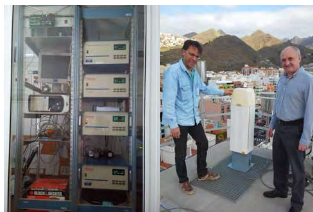
Figure 3.9. Air quality analyzers in the SCO Lab (left), and Ramón Ramos and Pedro Miguel Romero (right) with the Vaisala CL51 ceilometer on the SCO terrace.
