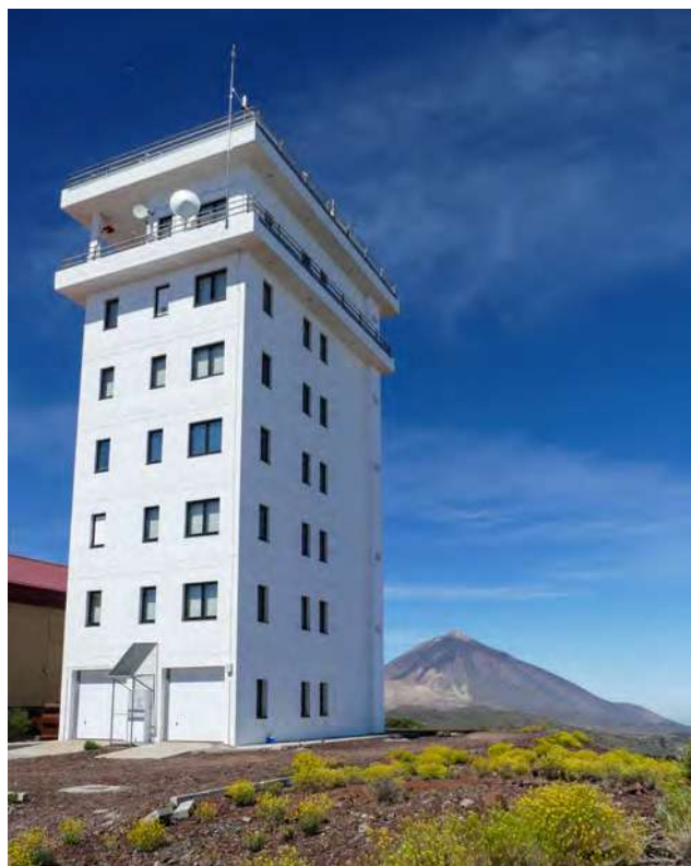
Figure 3.7. Images of IZO Instrument terrace and technical tower.
