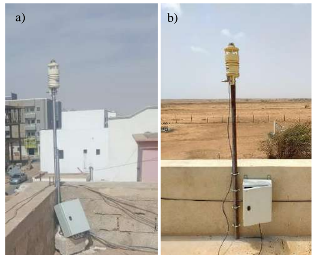
Figure 17.9. PM 10 data/PM-LCS installation at a) Mauritania and b) Isla de Sal (Cape Verde).
