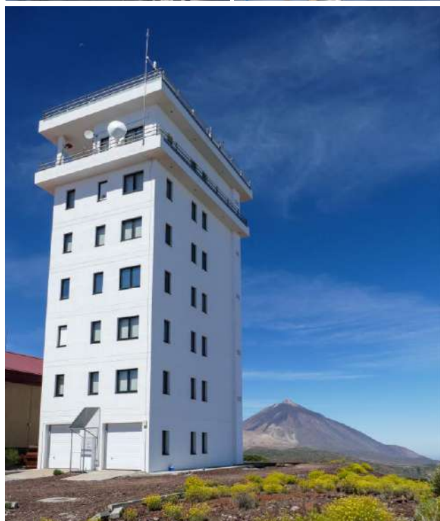
Figure 3.9. Images of IZO Instrument terrace and technical tower.
