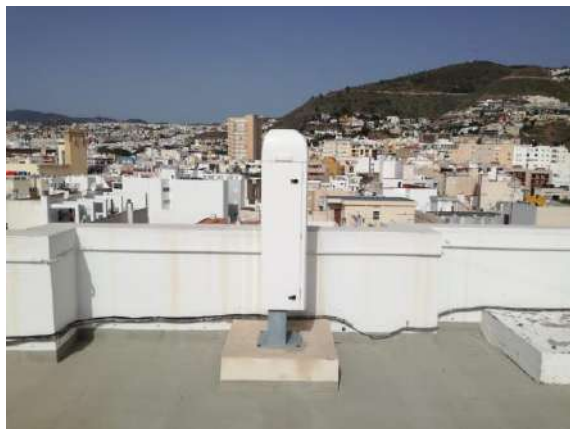
Figure 9.5. CL51 ceilometer in operation in SCO.
