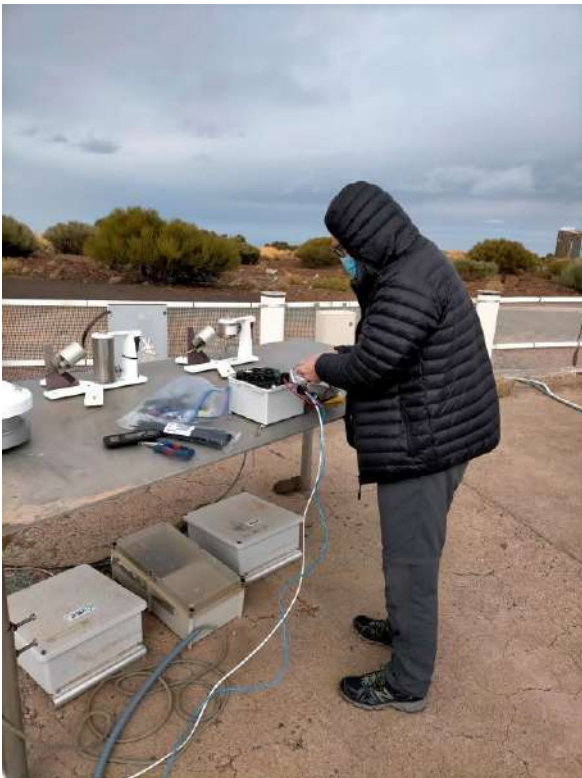
Figure 19.2. Dr Martin Aubé at Izaña during the installation of the new CoSQM version 2 instrument in November 2021.
