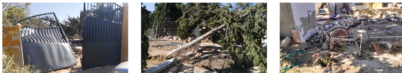
Fig. 11. Damages created by Tornado 2 (Jiménez Alonso et al., 2020). From left to right: metallic entrance door, damaged trees and fences, and construction materials and tools.
