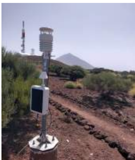
Figure 20.3. PM-LCS installation at IARC (CREWS DUST sensors)
